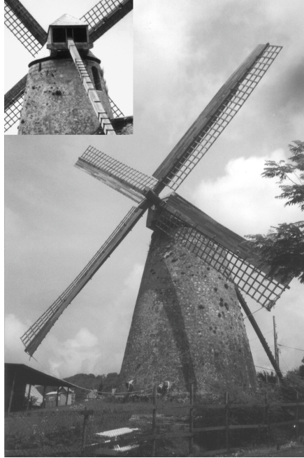
FIGURE 2.2. Morgan Lewis windmill, Barbados. The blades move a mechanism used to smash sugar canes. Built in 1727, it shows some technical solutions (yaw control and twisted blades) applied in order to improve its performance.
