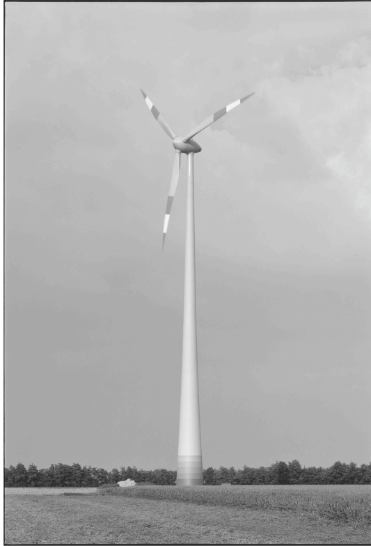
FIGURE 1.2. Enercon E66. Courtesy of Enercon GmbH.
